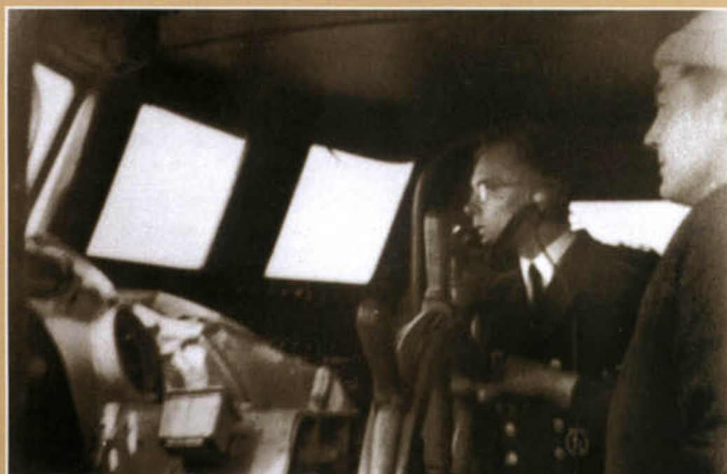
Below: On the bridge of the S105, the officer in the background is radioing the engine room to give instructions to the Chief Machinist who can immediately change the boat's speed.
