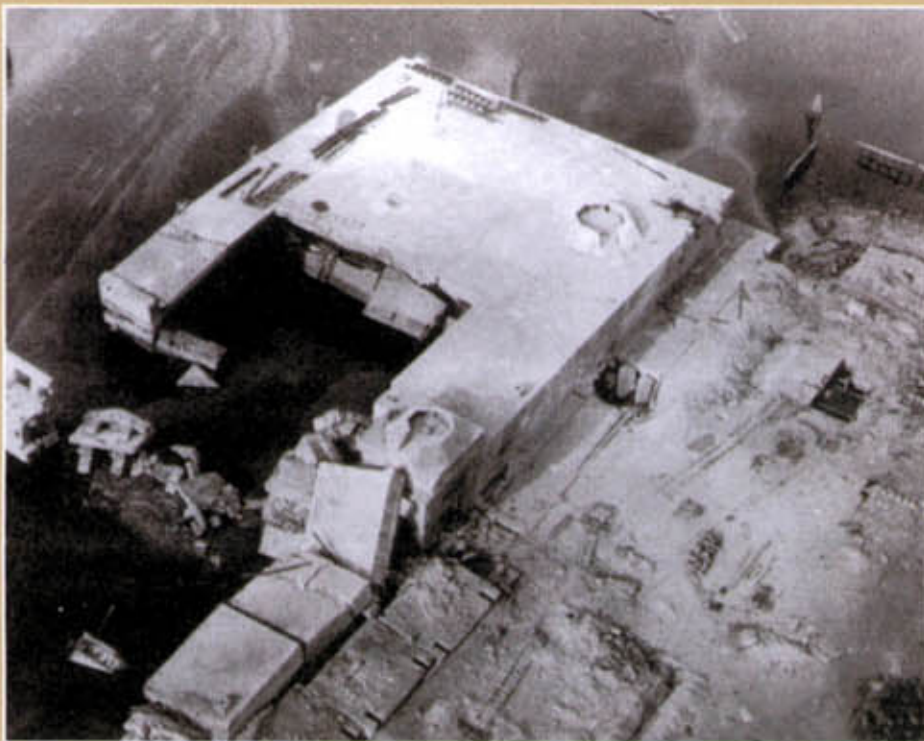
Above and left: The result of the explosion of two Tallboys on the upper structures of the S-Bunkers in Le Havre. Part of the concrete roof has caved in on the boats docked underneath.
