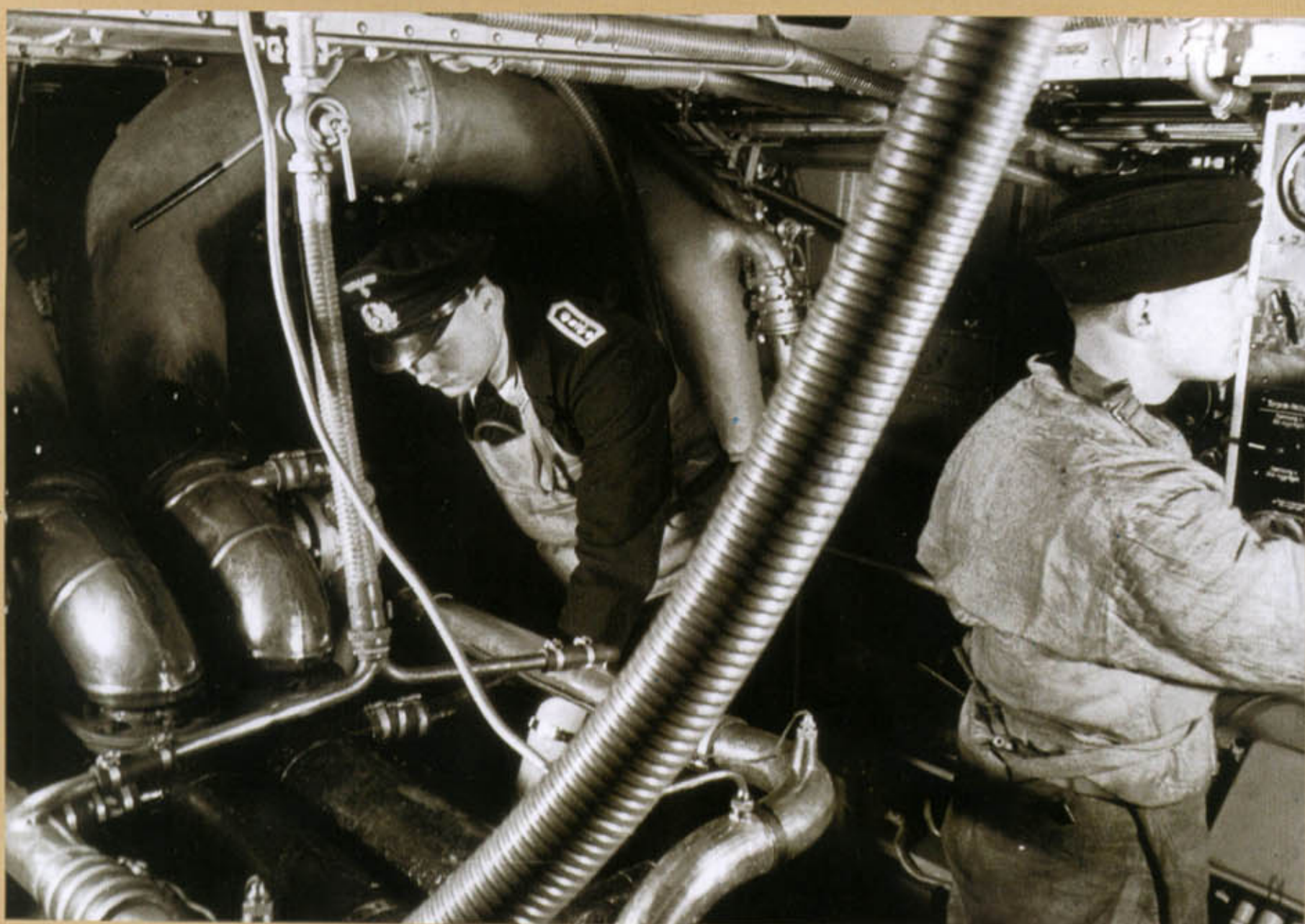
Below, and next page: In the machine room of an S-Boote on operations. The speed of the three diesel engines was under constant surveillance throughout the mission. If one engine broke down, the two other working engines were capable of getting the boat back to her home base.
