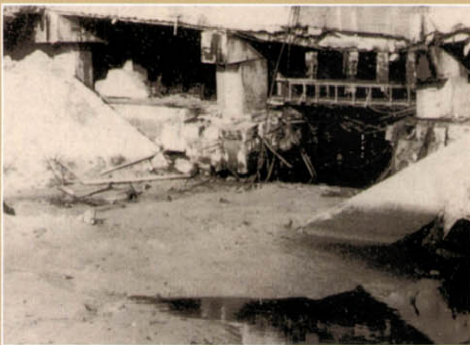
Centre: The IJmuiden S-Bunker after the air raid launched by the Bomber Command Squadron 617 aircraft on December 15, 1944. Two 5.5-ton Tallboys penetrated inside the building, destroying the S198 and damaging the S193, S195 and S701. In less than ten minutes the entire 8th flotilla was out of action.
