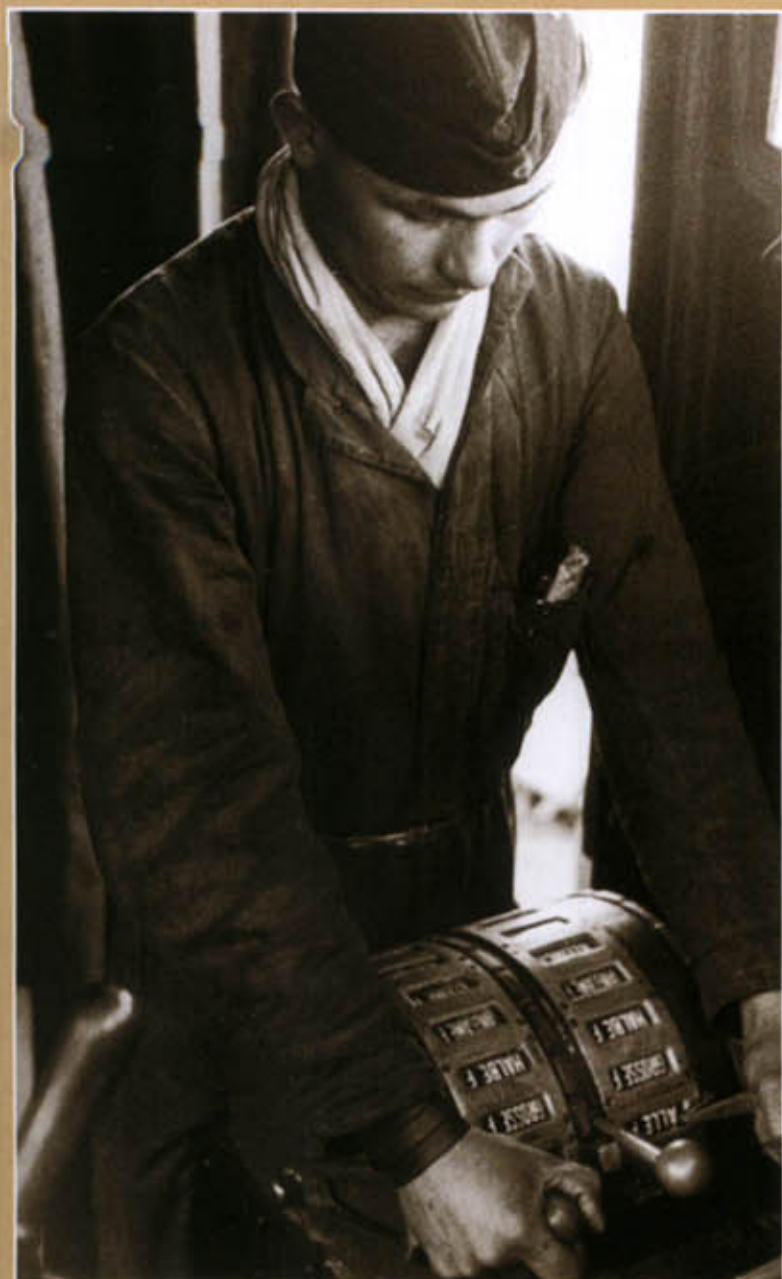
Left: In the command post of an S-Boote on operation. A crewman is pulling one of the three « Chadburn » levers ; the Chadburn box transmitted orders concerning engine speed to the engine room. The chief machinist received information through an identical apparatus installed in the engine room about the desired speed to be applied to the three boat engines.
