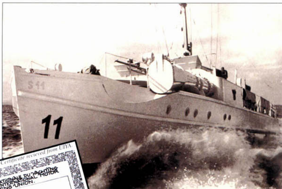
Above: The S11 training in the Baltic Sea. This snapshot, reproduced from a post card, was taken before the beginning of the war. This unit was part of the S10-S13 series, delivered in 1934. She was propelled by three 1200-hp MB 502 engines allowing her to reach a top speed of 35 knots. The S11 was turned over to the Soviet Navy in November, 1945.
